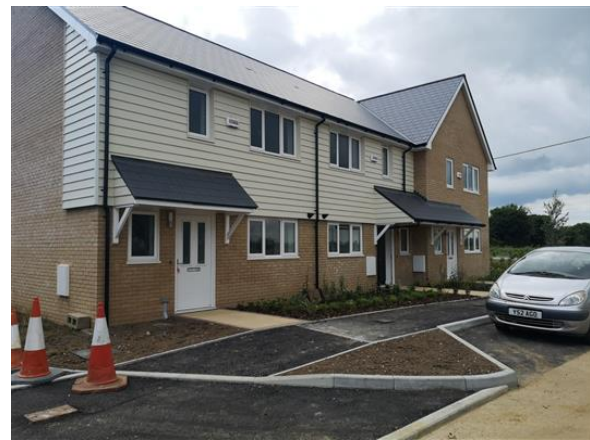
Affordable housing at George Close, Capel le Ferne
